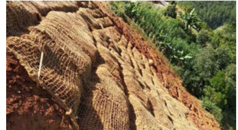
Slope Treatment with coconet
